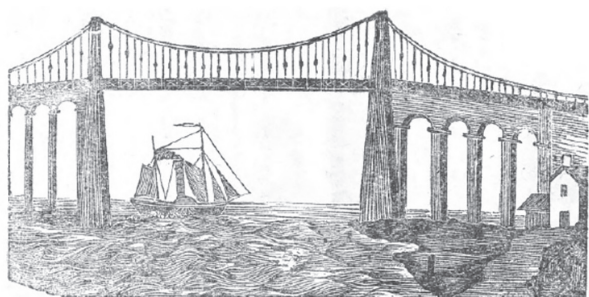
Menai suspension bridge (from [1]).
