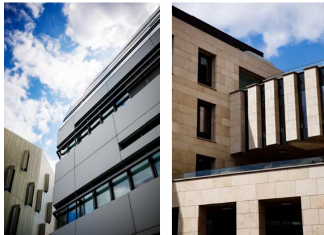
Lab Buildings East (left) and West (right). The Institute of Science and Technology Austria (ISTA) offers state-of-the-art research facilities and scientific support units in all major disciplines. © Peter Rigaud/ISTA
