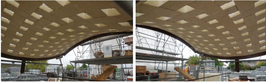
Figure 3. Pictures of a saddle vault with Abeille’s bonding built in Troyes (France), 2013 [20].
