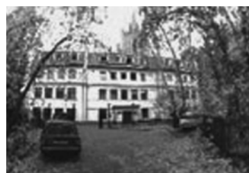
The newly reconstructed MCCME-IUM building
