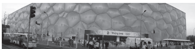
Figure 3a: The Beijing Olympics Swimming Cube, where Michael Phelps earned his gold, used a soap bubble cluster model.
